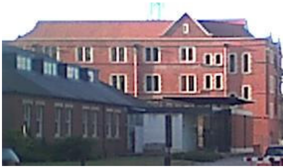
The 'Ark' cleaned and restored with the new gable, seen in the early morning sunlight.
