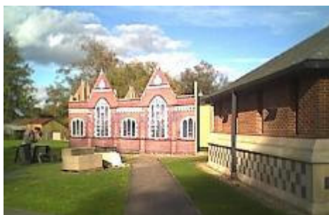
The 'folly' under erection.
