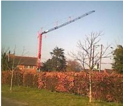
The crane seen from the park
