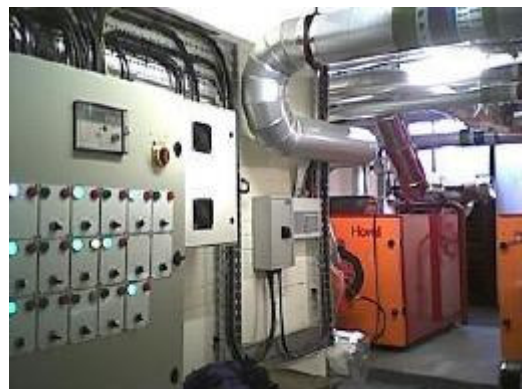
The refurbished boiler room
