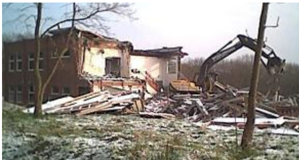
Ditcham block in course of demolition
